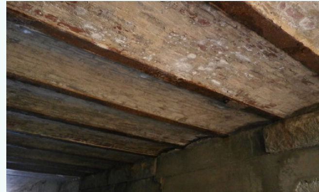
Underside of 1898 jack arch bridge (NHDOT)
