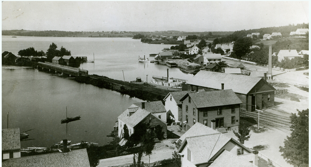
1880s view facing northeast, showing the earlier Lakeport railroad bridge with a wooden boxed pony truss bridge over the water (Laconia Public Library)
